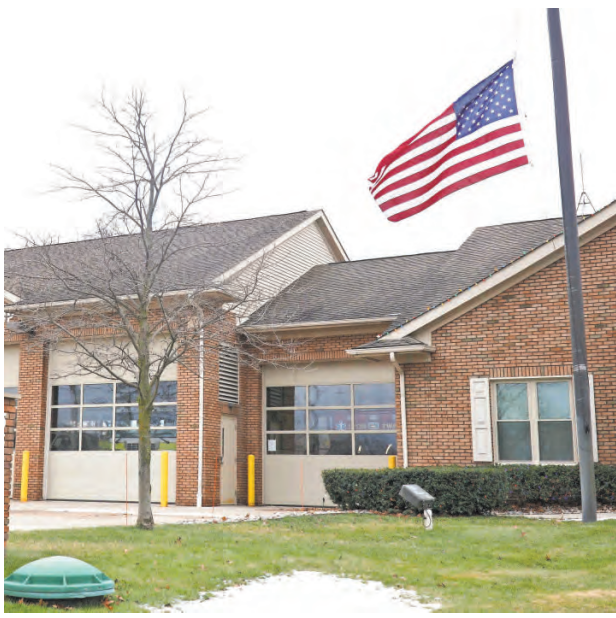
Lyon Township's Fire Station No. 2 sits along Ten Mile Road near Milford Road. JOHN HEIDER/HOMETOWNLIFE.COM
